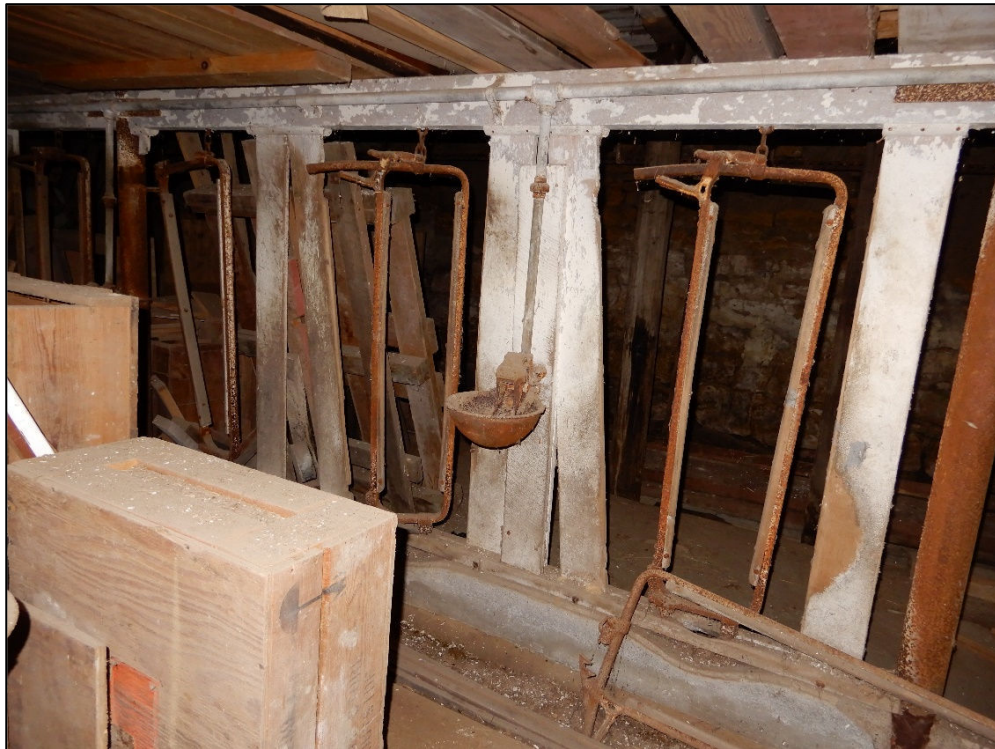
Figure 13. Detail of milking stanchions and watering poles in basement level of Banked Barn looking NNW. Photograph taken by Tallgrass, October 1, 2019.
