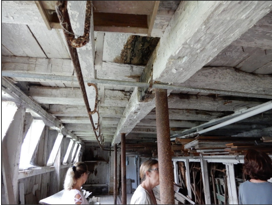
Figure 15. Interior of basement-level of Banked Barn looking West. Note metal poles supporting hand-hewn beams in what would have been the original forebay. Photograph taken by Tallgrass, October 1, 2019.
