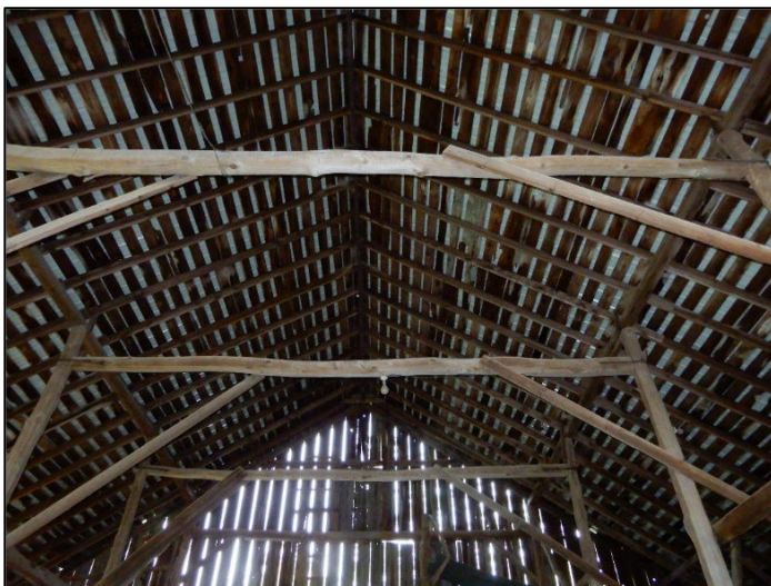
Figure 28. Interior of Feeder/Hay Barn looking West in the north bay of the barn (left); and bents in the center aisle formed of poles nailed and bolted together with metal straps looking West (right). Photographs taken by Tallgrass, October 1, 2019.
