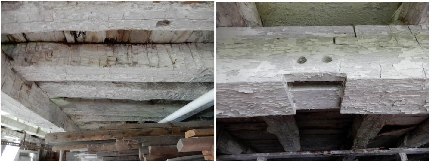
Figure 11. Detail of hewn cross beams in ceiling of basement level of Banked Barn of area where original forebay was enclosed and open to the interior removing some vertical posts in the process. Photographs taken by Tallgrass, October 1, 2019.
