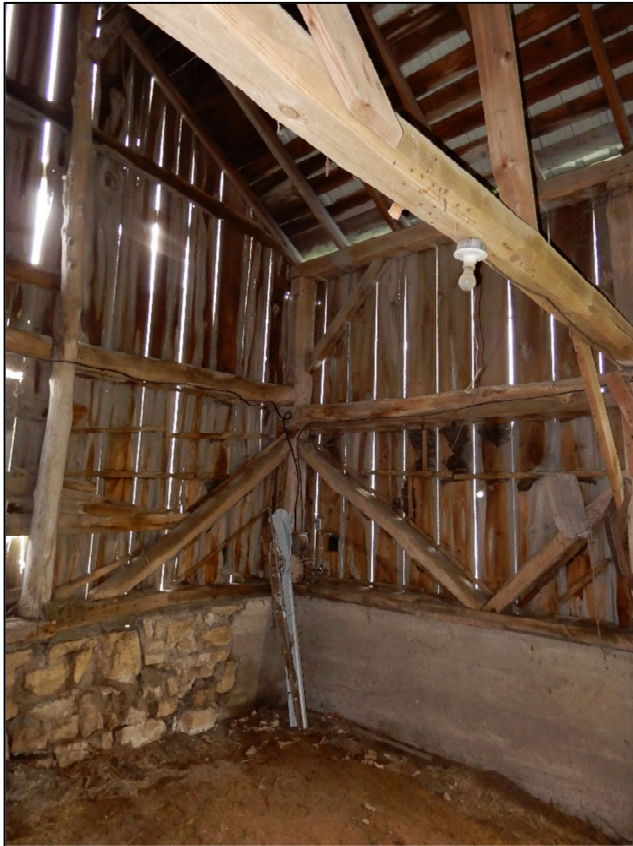
Figure 29. Interior of Feeder/Hay Barn showing (Left) the junction of the exterior stone foundation with the concrete foundation in the SE corner of the barn and (Right) a detail of the pole/post framing showing the cross-beam poles attached to the vertical square posts with nails and metal straps. Photographs by Tallgrass, October 1, 2019.
