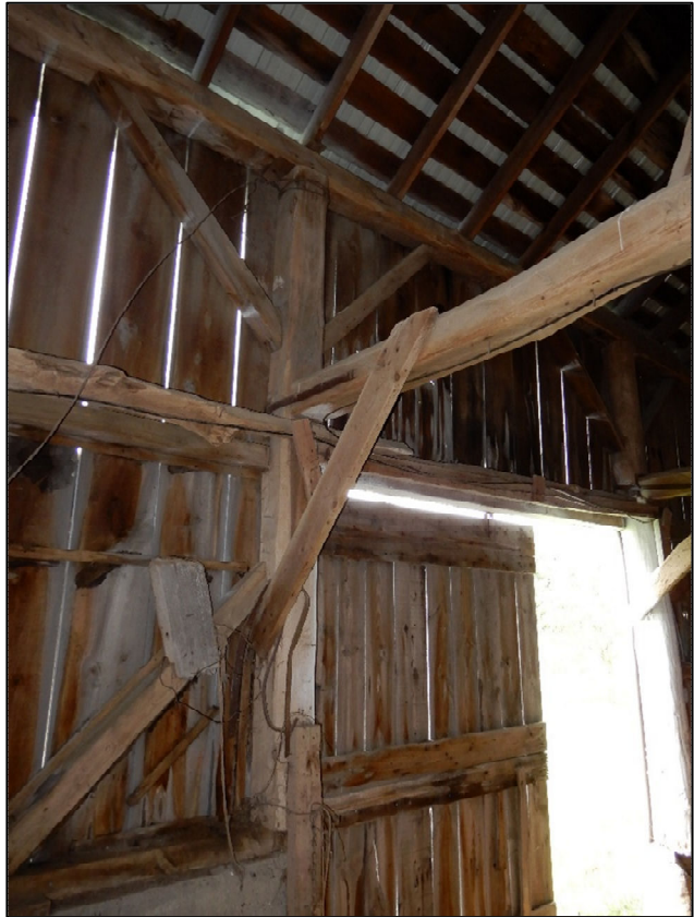
Figure 29. Interior of Feeder/Hay Barn showing (Left) the junction of the exterior stone foundation with the concrete foundation in the SE corner of the barn and (Right) a detail of the pole/post framing showing the cross-beam poles attached to the vertical square posts with nails and metal straps. Photographs by Tallgrass, October 1, 2019.
