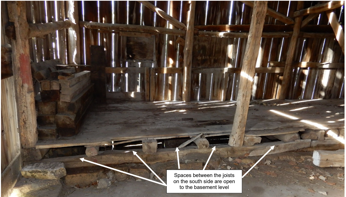
Figure 31. Detail of wooden plank floor on south side of Crib/Hog House looking ESE showing the open spaces between the floor and the hewn joists that allowed for additional air flow into the basement level. Note the light visible in the basement level that would have fully lit when the doors were opened. Currently the doors are nailed shut. Photograph taken by Tallgrass, July 22, 2020.
