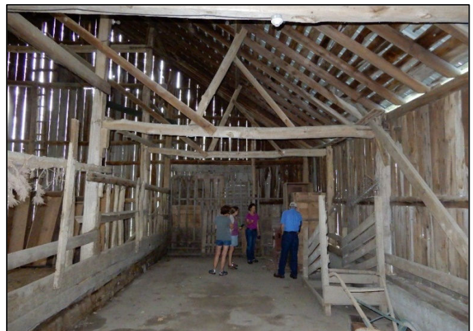
Figure 28. Interior of Feeder/Hay Barn looking West in the north bay of the barn (left); and bents in the center aisle formed of poles nailed and bolted together with metal straps looking West (right). Photographs taken by Tallgrass, October 1, 2019.
