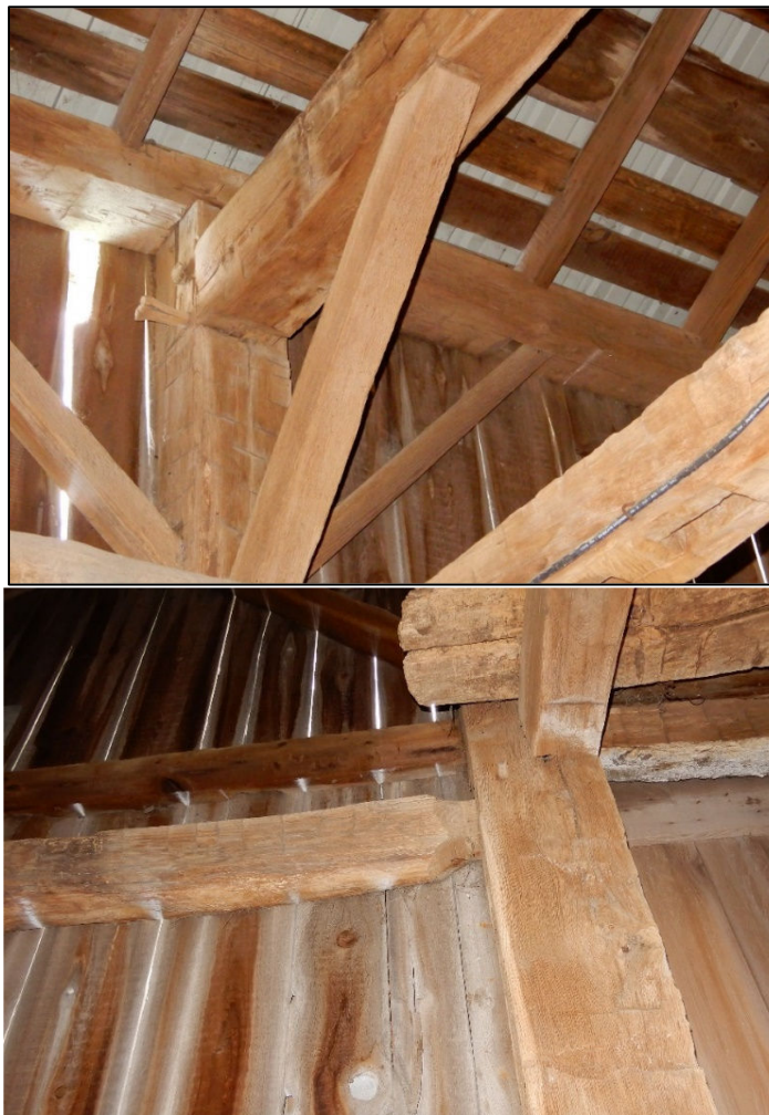
Figure 18. Top: Detail of hand-hewn posts and beams, sawn angled bracing, and the mortise-and-tenon, pegged joiner in the upper loft framing of the Banked Barn; Bottom: Detail of hewn joinery of loft wall framing in the Banked Barn looking up. Photographs taken by Tallgrass, October 1, 2019.
