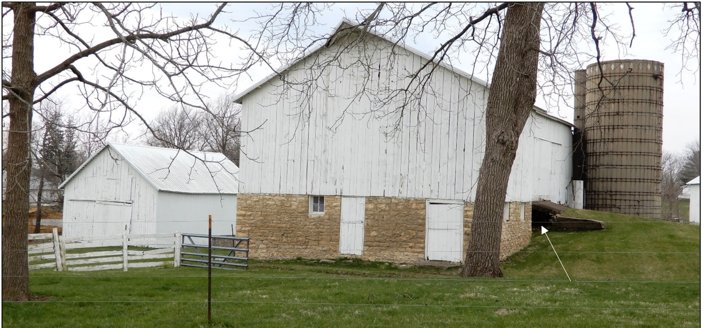
Figure 4. Barn looking WSW and showing the north side banked into the slope, with the earthen ramp having concrete side walls and a concrete bridge connecting the ramp to the north centered door on the upper level of the barn. White arrow is pointing to the open space under the concrete bridge. Photograph taken by Tallgrass Archaeology LLC, April 11, 2020.
