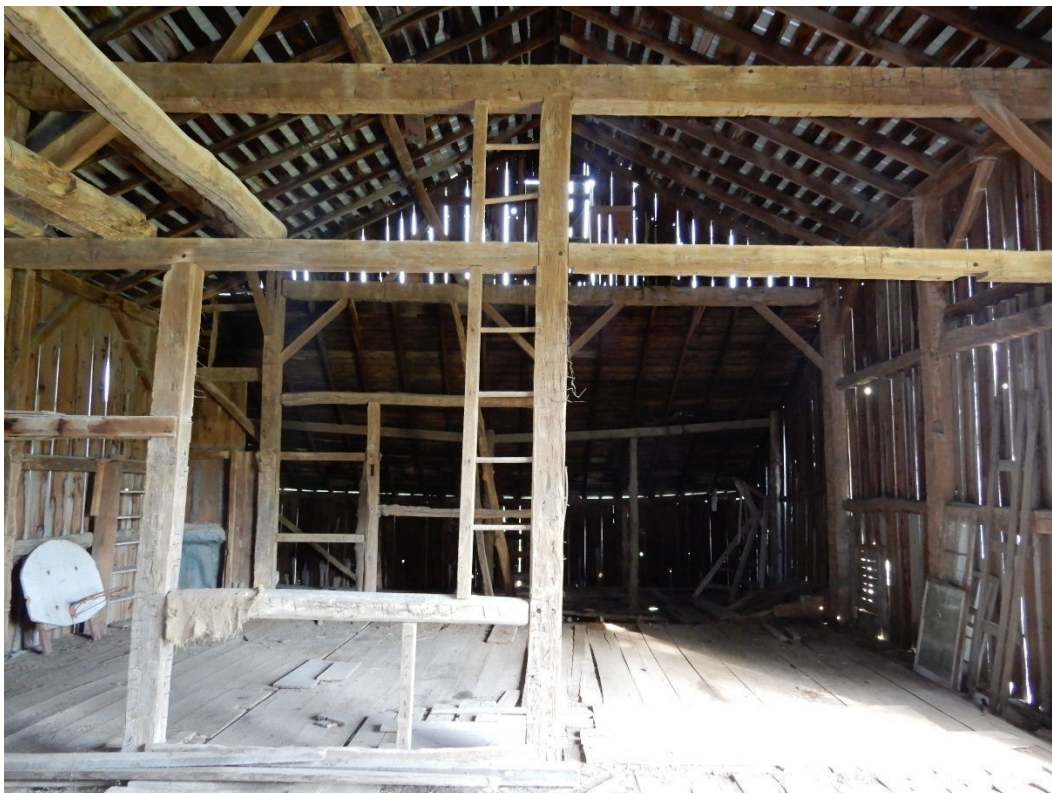
Figure 20. Interior and end wall loft framing of west half of Banked Barn looking west into the shed-roofed addition. Photograph taken by Tallgrass, July 22, 2020.
