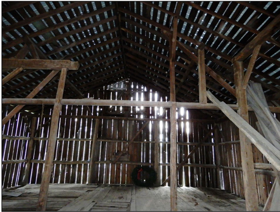
Figure 19. Interior bent framing of loft area of Banked Barn looking East. Note that some original members are missing likely from the 1908 tornado that took off the roof of this building. Photograph taken by Tallgrass, October 1, 2019.
