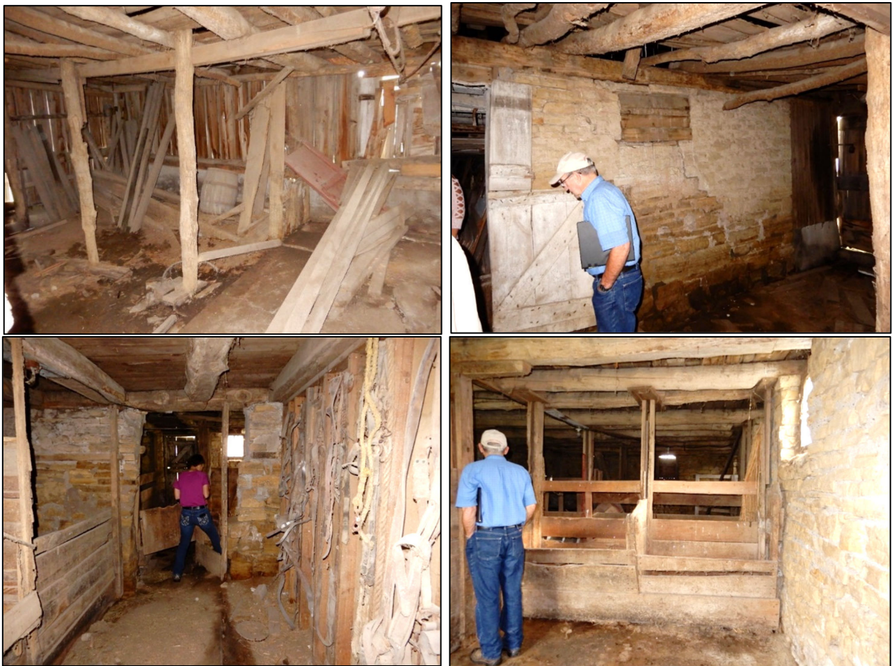
Figure 17. Clockwise from top left: Interior of west shed addition to gable end of Banked/Basement Barn looking WSW; interior of west shed addition to Banked/Basement Barn showing original exterior of west foundation wall of barn; interior of east addition looking north at stalls and wooden feed bunks; and door cut into east wall of original stone foundation for access into east addition and showing tack hanging on the aisle wall. Photographs taken by Tallgrass, October 1, 2019.
